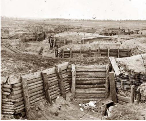
Well-established trenches, showing logs used to shore up the walls.
