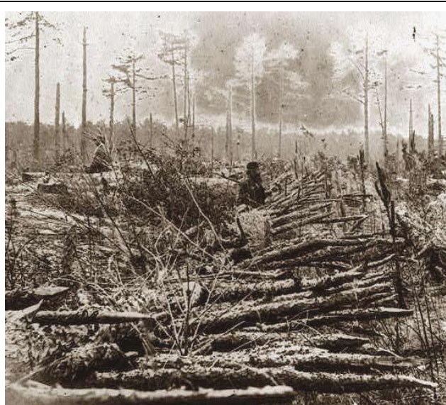
An abatis of sharpened stakes embedded in the embankment of a ditch.
