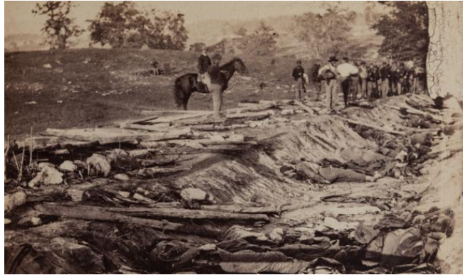
A rifle-pit, seen after the action has ended. Note the piles of rocks and rails to the front.
