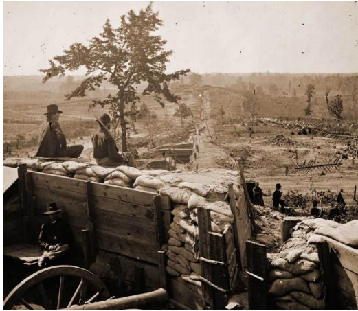
A heavily fortified position, showing planks shoring up a trench of earth and sand-bags. Note the chevaux-de-frise in front of the position.
